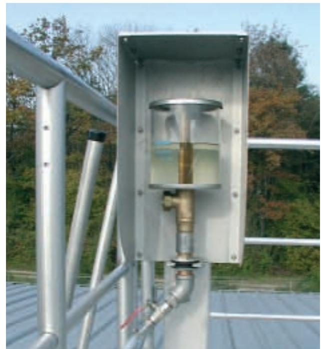
Leak control for VRM® bearing
