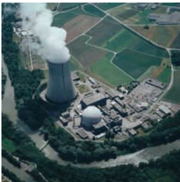
Aerial photo of the nuclear power plant Gösgen
