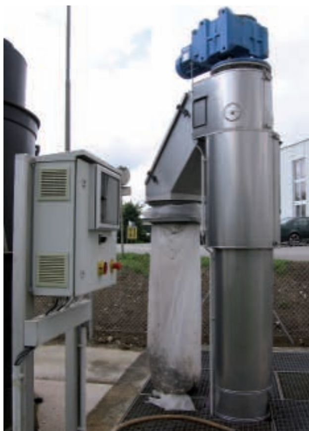
HUBER ROTAMAT® Pumping Stations Screen RoK 4-700-3 with insulation
