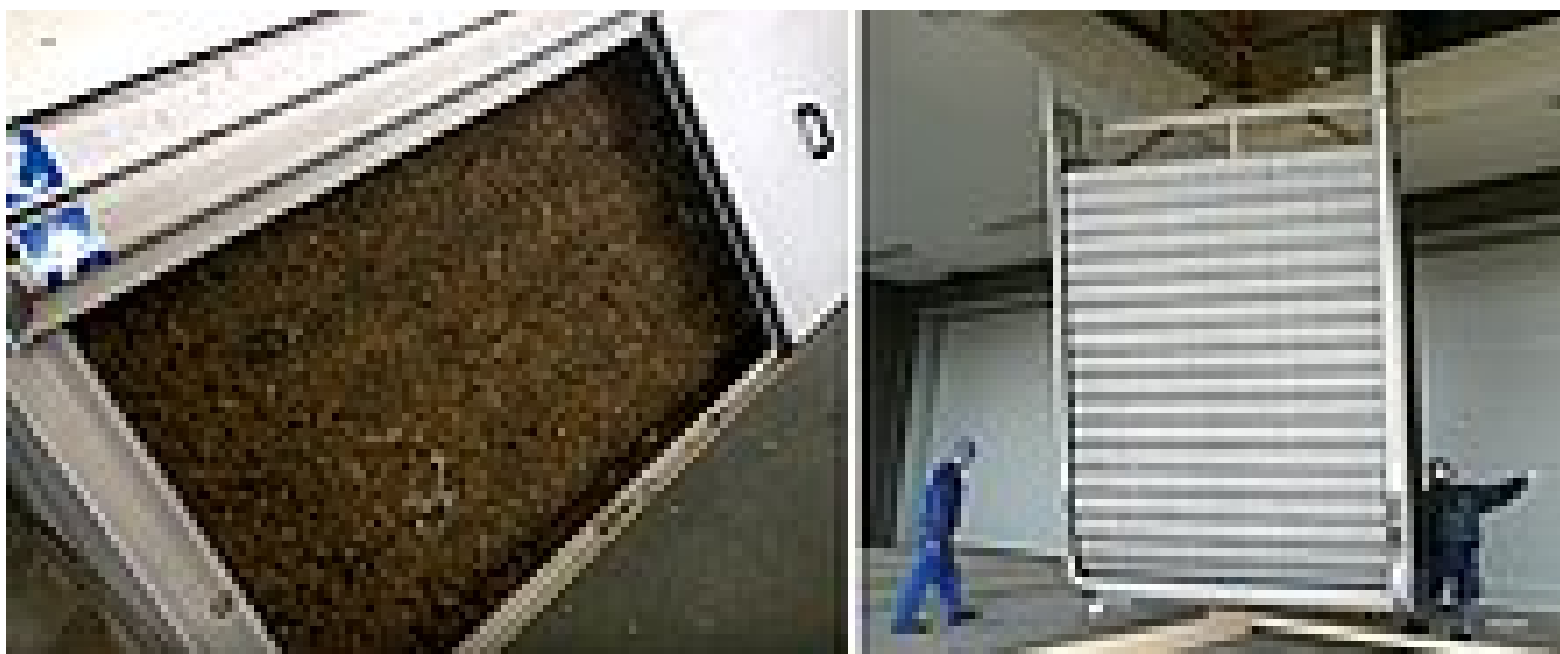
HUBER Belt Screen EscaMax®: Blinding of the screen during load operation and insertion of the bottom part of a two-part HUBER EscaMax® screen into the screen building
