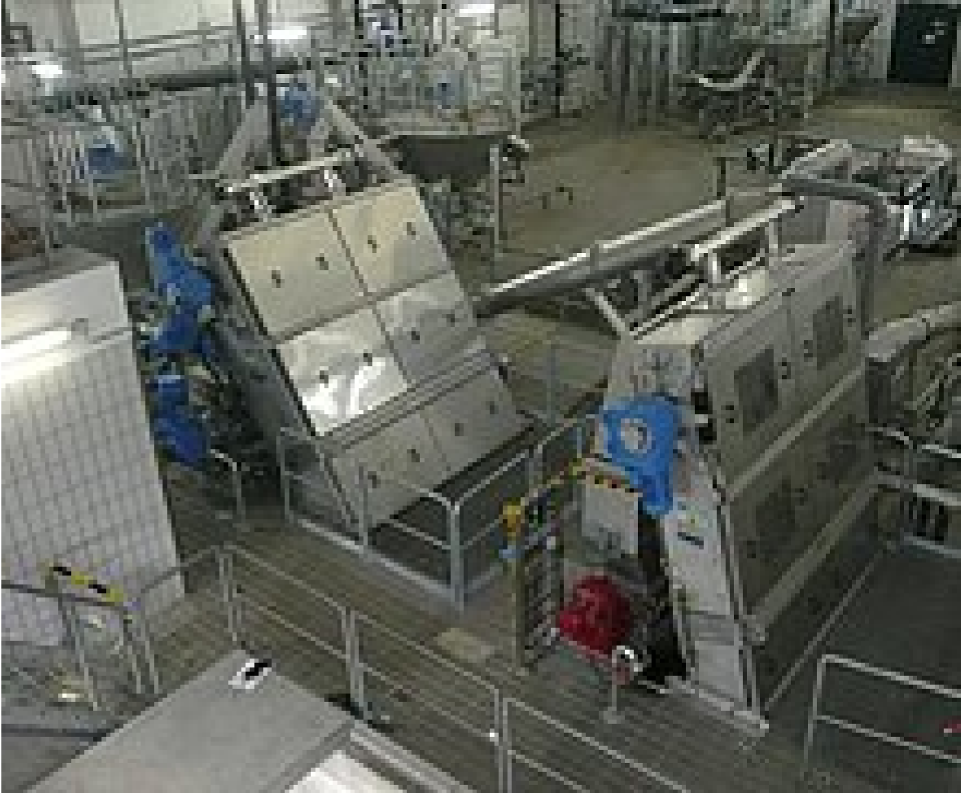
Line 1 shortly after start-up
