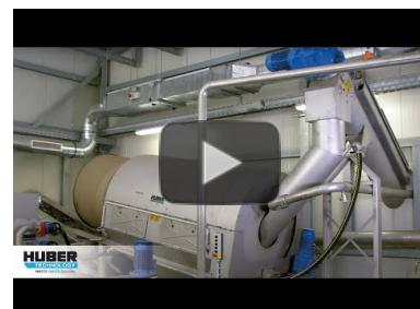
Video: HUBER Rotary Drum Fine Screen ROTAMAT® Ro2 in a grit treatment process for wash-out of organics
