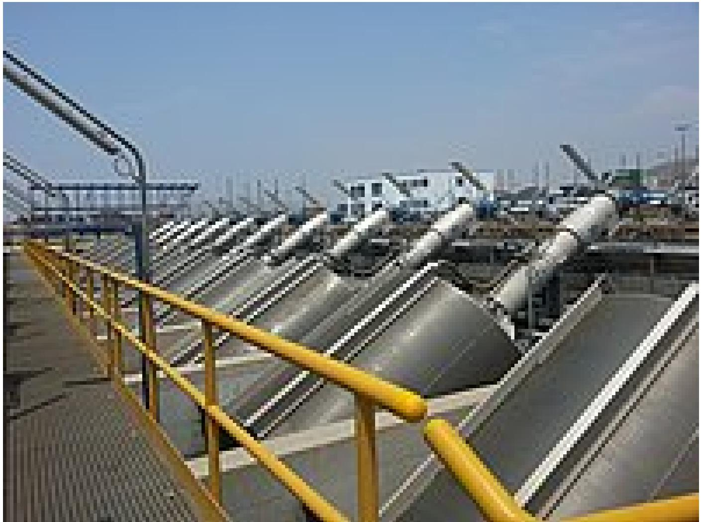
Reliable and well-proven inlet screen for municipal sewage treatment plants and industrial wastewater and process water screening
