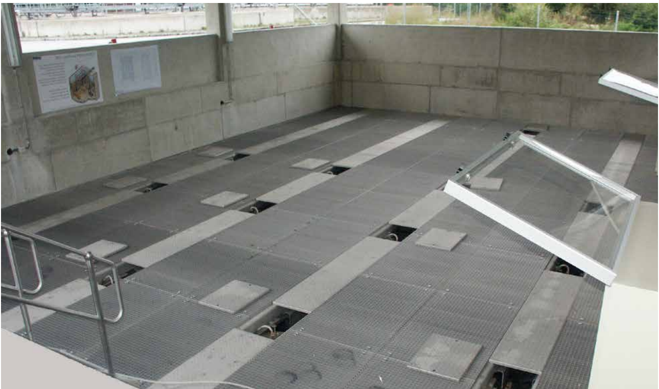
HUBER Active Carbon Filter CONTIFLOW® GAK (tank design).
