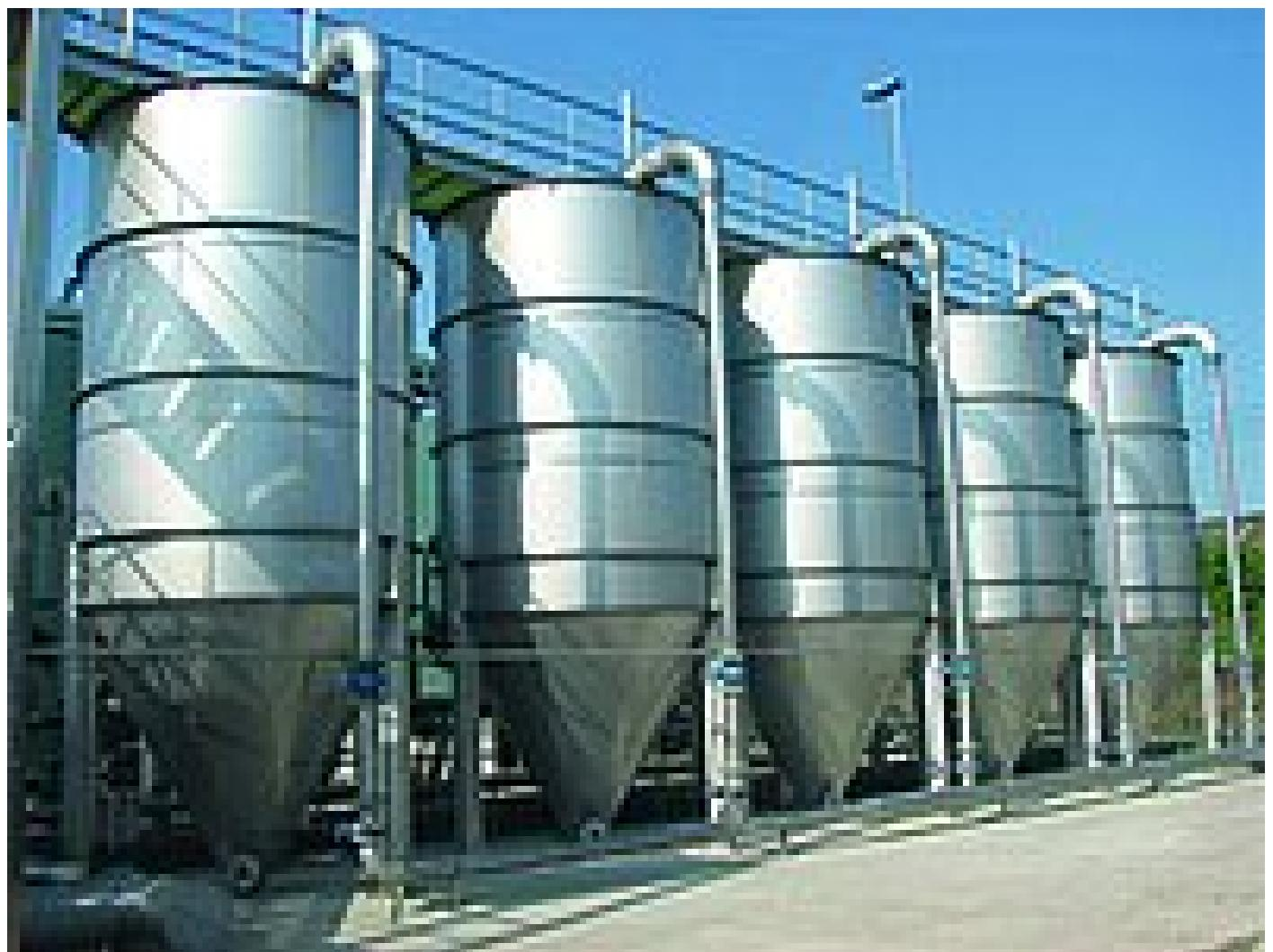
The HUBER Active Carbon Filter CONTIFLOW® GAK removes micropollutants from the wastewater flow. The system uses granulated active carbon and is installed downstream of the secondary clarifier. An important advantage of the HUBER Active Carbon Filter CONTIFLOW® GAC is that it has no influence on existing process-engineering systems on the sewage treatment plant and can be optimised further by adding a sandfilter or an upstream ozonisation plant.
